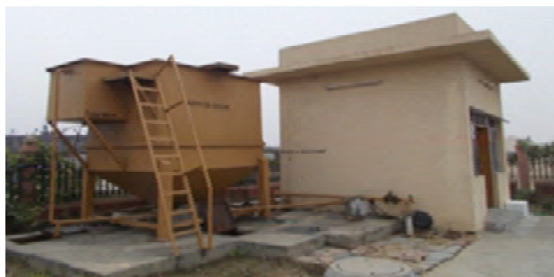
Effluent treatment plant at CSIR-CDRI; Lucknow
