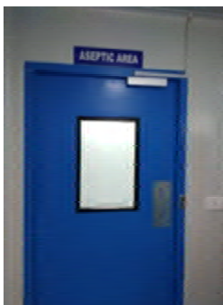
Views of the manufacturing area, awaiting final commissioning as on date of reporting. Entrance to the manufacturing area is biometrically controlled. The main entrance to the facility (left) is a Class C foyer, leading to a Change Room where operators will don PPE to enter a Class B area. The room for Aseptic Processing (manufacture of injectables) is preceded by a Class B area. Class A conditions for the actual manufacturing operations will be achieved by the use of an isolator placed in the Aseptic Area (right).
