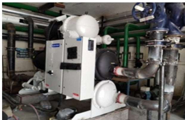
The new 200 TR HVAC chiller at the Old campus
